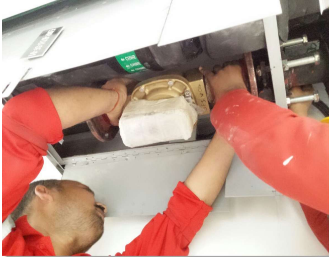
Figure 1-mounting the Smart-Actuator must be made by qualified personnel
