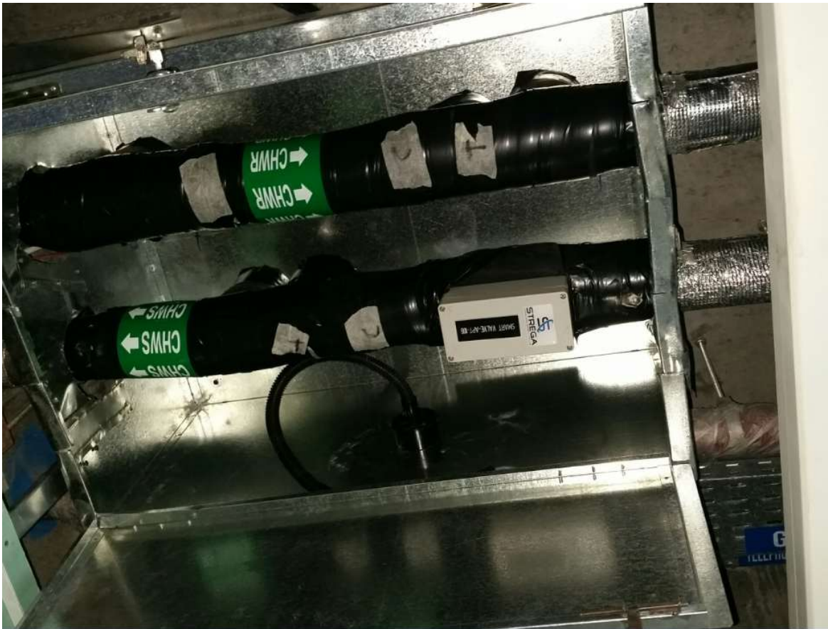
Installation of a Smart-Actuator in a ceiling cabinet
