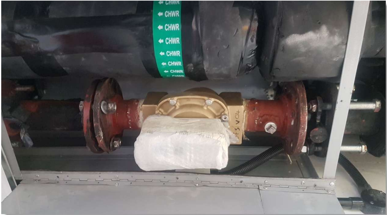
Large size pipe sections should use flanges (DN65 shown)
